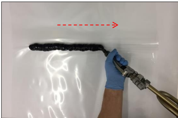
FIGURE 9 Apply the bead in the fold direction
