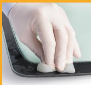
■ To remove contamination: wet Sika<sup>®</sup> Cleaner PCA with Sika<sup>®</sup> CleanGlass and rub the area
