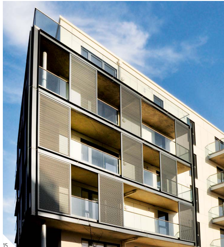
Threshold Residence, Parsons Green Project Participants Client: Threshold Housing Association Facade: Cladding UK
