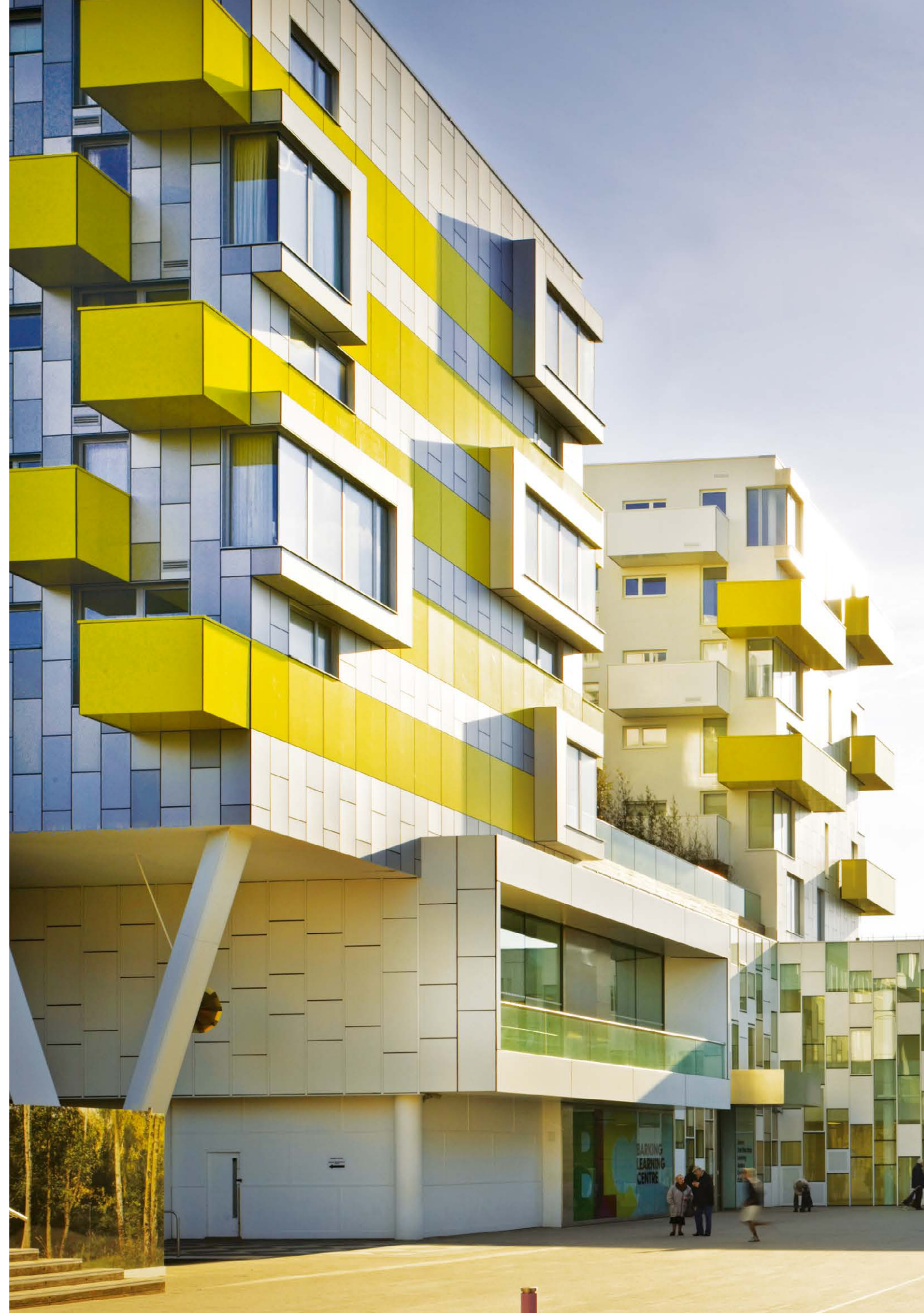
RIGHT, Project 148: Lifelong Learning Centre Barking Project Participants Architect: Allford Hall Monaghan Morris Facade: Cladding UK
