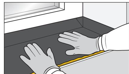
Membrane can be adjusted within 30 minutes after adhesive application.
