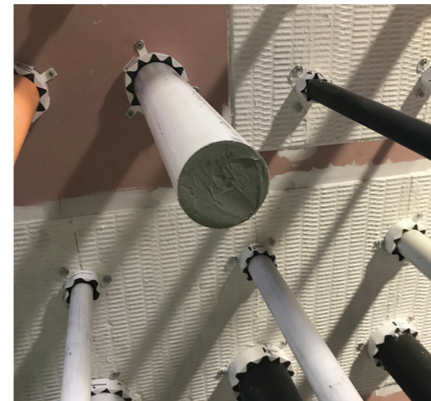
Pipe collars before ...
