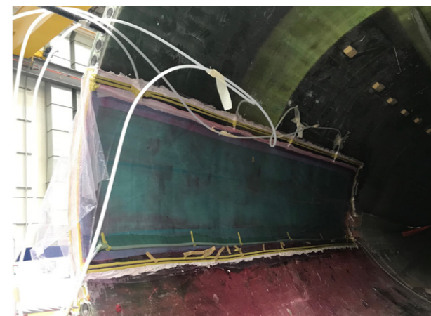
Overlamination of the root end bonding joint by infusion.
