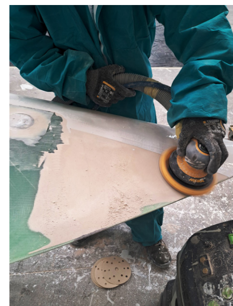
Grinding of a blade tip after applying the filler material SikaForce®-800 Red.
