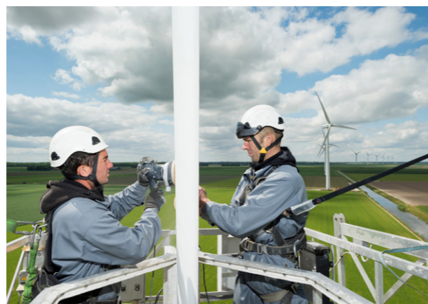
Repair technicians finishing a blade repair.
