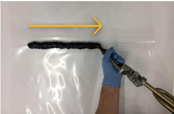
Figure 5: Apply the bead in the fold direction
