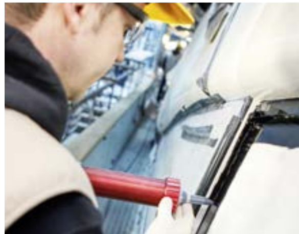
Adhesive application on the edging
