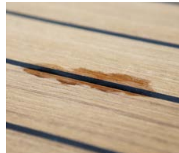
Teak deck damaged by water ingress
