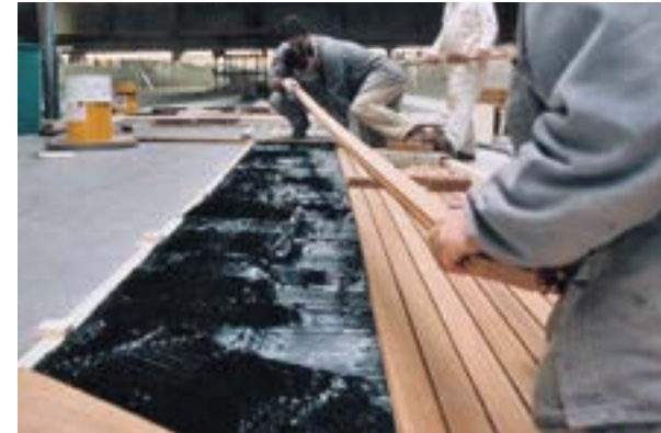
Application of deck
