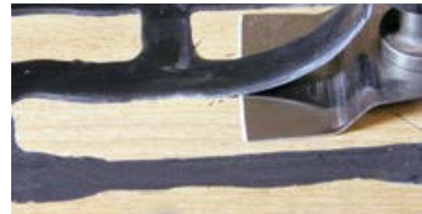
Remove excess 290 DC PRO with an oscillating scraper
