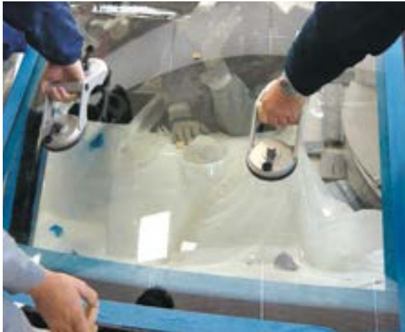
Inserting the window
