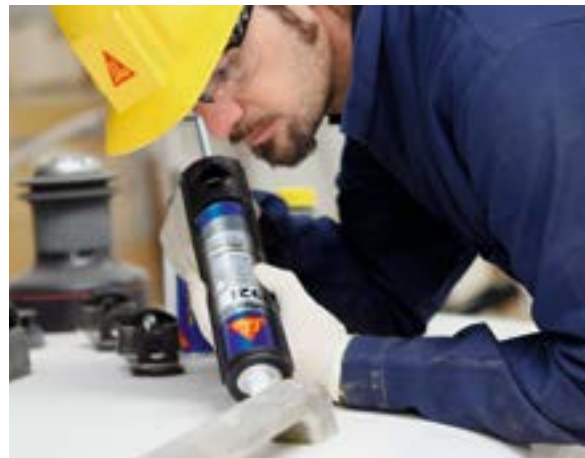
Bonding of the rub rail with Sikaflex®-292i
