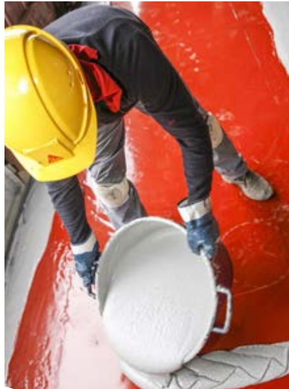
Pouring the mixed SikaTransfloor®-352 SL onto the deck
