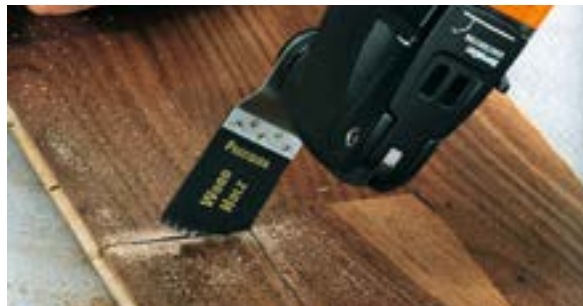
Cutting the strips with a vibrating saw
