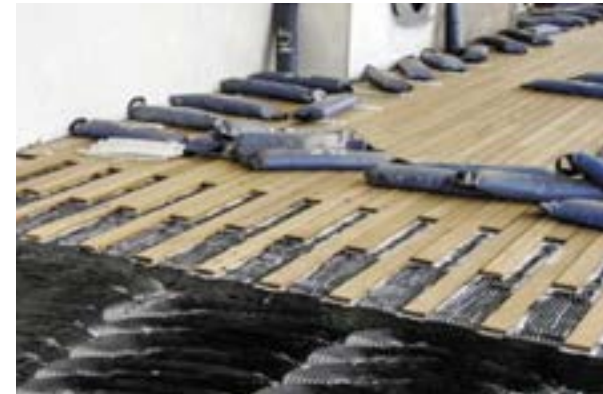
Teak strips embedded in Sikaflex®-298 and secured with weights
