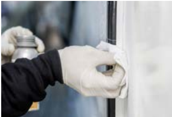
Pre-treatment of the ceramic screen-printed edge with Sika Aktivator-100
