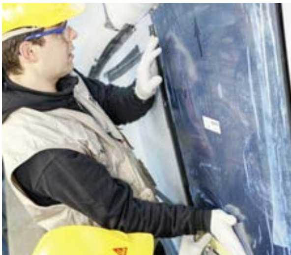
The window can still be aligned immediately after joining
