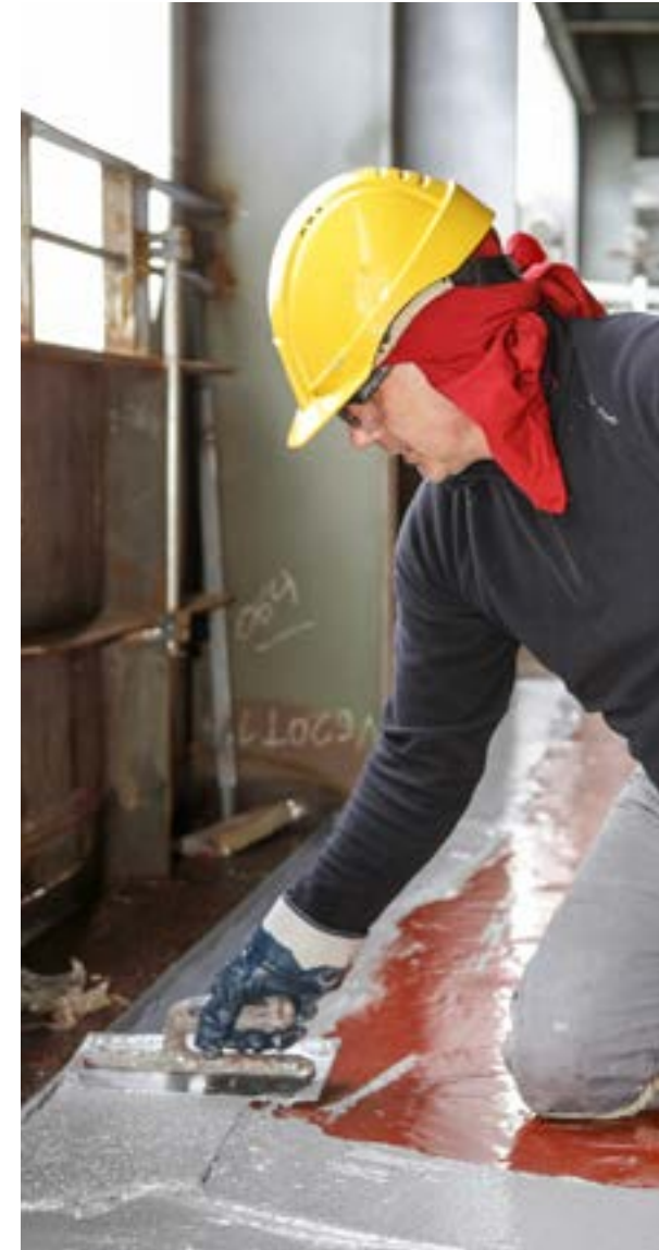
Spreading SikaTransfloor®-352 SL with a spatula
