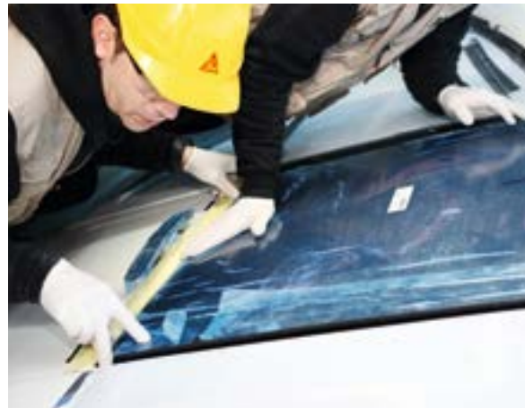
Application of Sikaflex®-296
