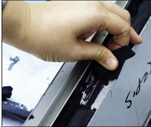
Figure 27: Adhesive failure, deglazing test negative
