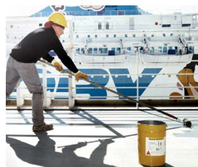
Fig. 3 Applying SikaCor® ZP Primer with a roller
