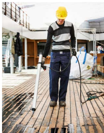
Fig. 17 Applying Sikaflex®-290 DC PRO
