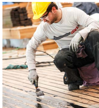
Fig. 19 Compressing Sikaflex®-290 DC PRO with a spatula
