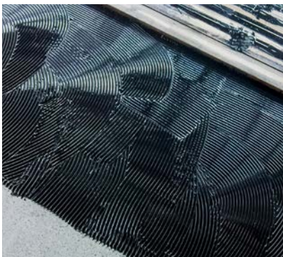
Fig. 12 Sikaflex®-298 applied with a comb spreader
