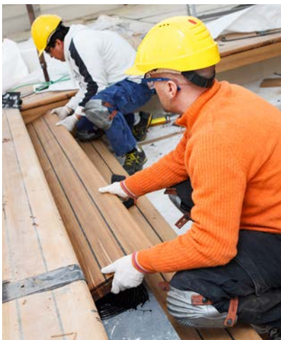
Fig. 13 Putting down the decking
