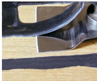
Fig. 49 Picture Removal overstanding Sikaflex®-290 DC PRO with a vibrating scraper power tool
