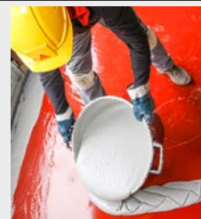
Fig. 7 Pouring the SikaTransfloor®-352 (SL/ST) to the floor
