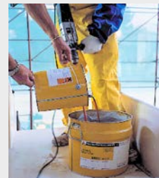
Fig. 6 Transferring the SikaTransfloor®-352 (SL/ST) to another container
