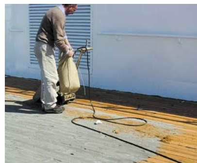
Fig. 20 Sanding the deck
