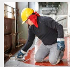
Fig. 8 Spreading the SikaTransfloor®-352 (SL/ST)
