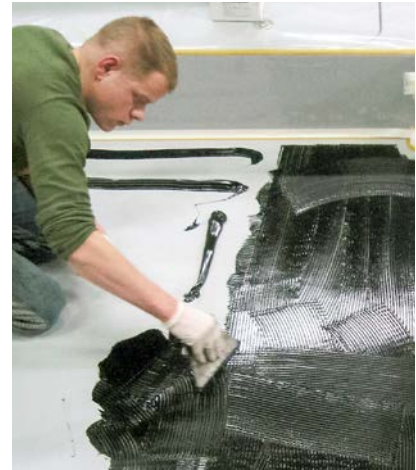
Fig. 55 Application of Sikaflex®-298
