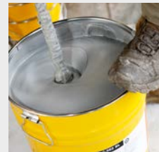
Fig. 5 Mixing SikaTransfloor®-352
