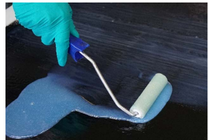
Roller application of SikaBiresin CR169 thix
