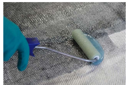
Wet lay-up with SikaBiresin CR168
